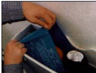
2. Place open end of Hippo over cistern float then turn over and fully immerse in water
