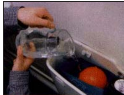
3. Flush toilet in normal manner whilst simultaneously pouring about 4 ℓ of water into Hippo
