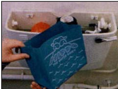
1. Put both hands inside the Hippo and push out corners to a box shape
